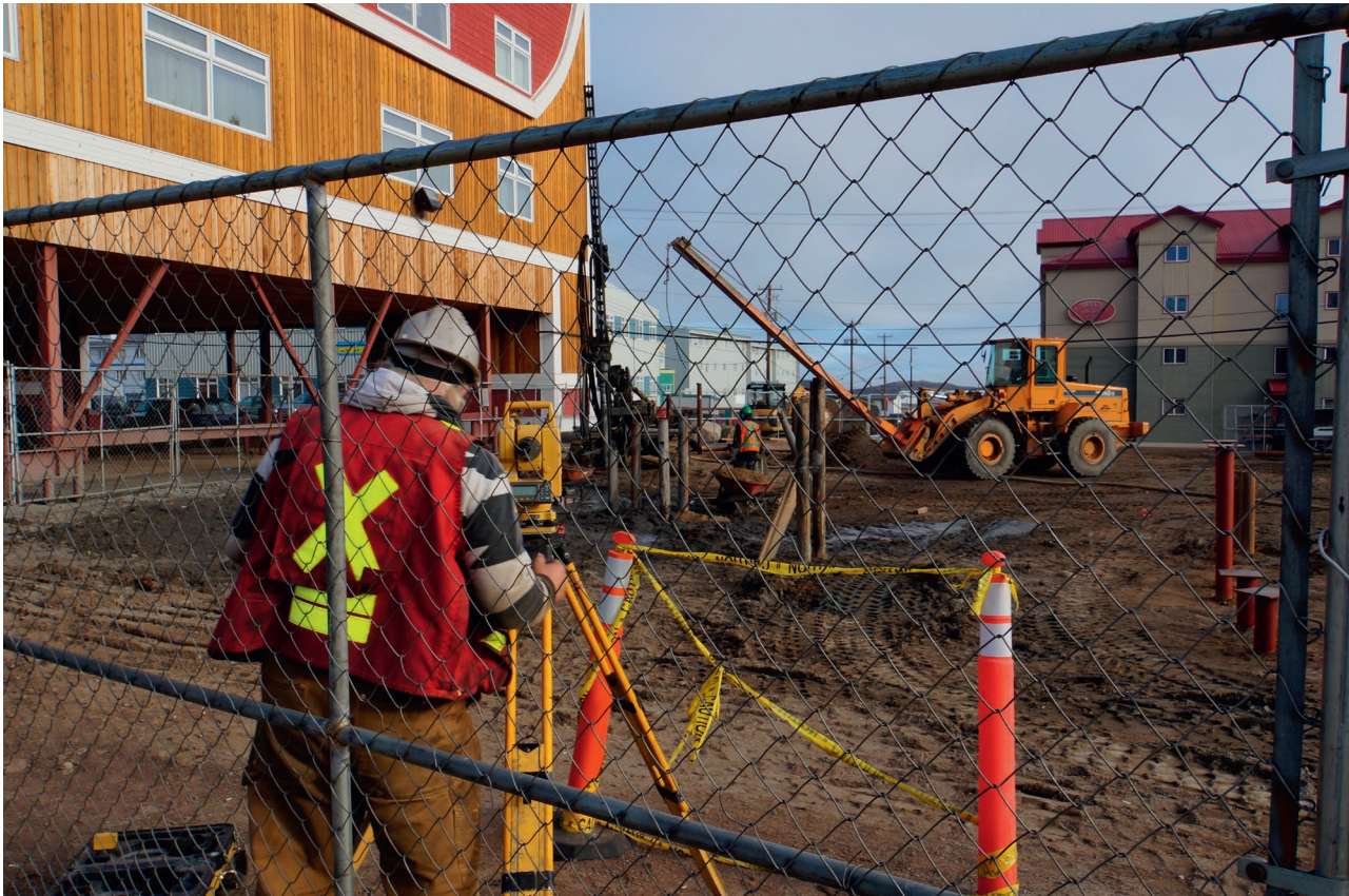
Figure 3 Iqaluit construction: driving pilings (the author)
