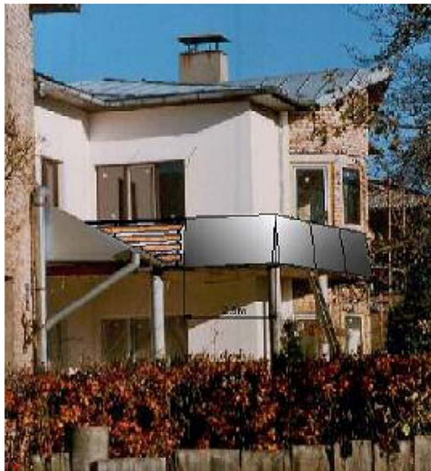
Figure 11. Lateral view – after installation (collector tilt 80^{\circ} , length \approx 2.5\text{m} , height \approx 1.16\text{m} )
