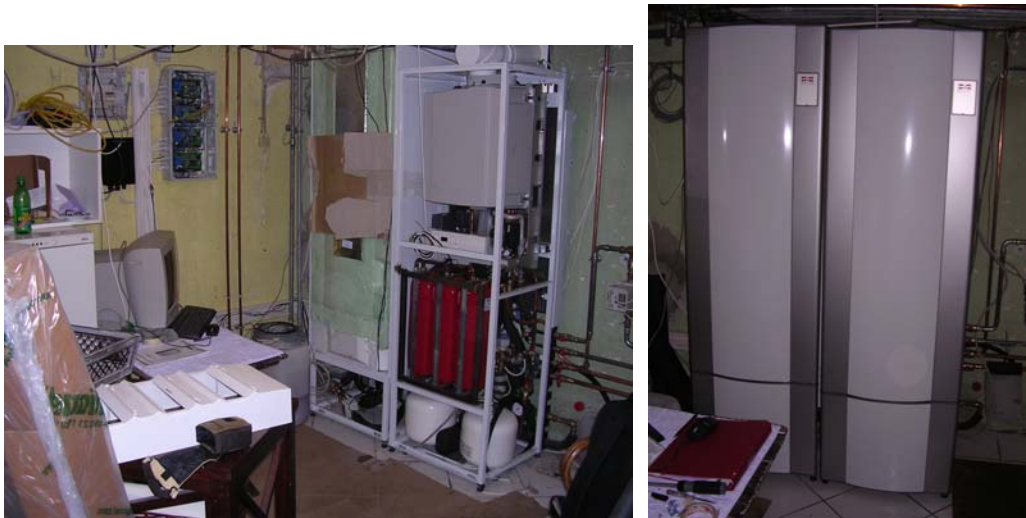
Fig. 8 Installation of the complete system before (left) and after (right) installing the cover plates.
