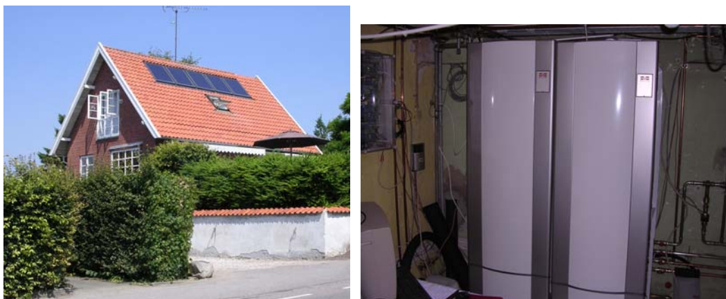
Fig. 21 Demonstration house with the collectors mounted on the roof (left) and the installed solar tank unit and the technical unit in the basement (right).
