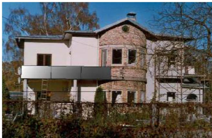
Figure 10. Front view – after installation (collector tilt 80^{\circ} , length \approx 6.5\text{m} and height \approx 1.16\text{m} )
