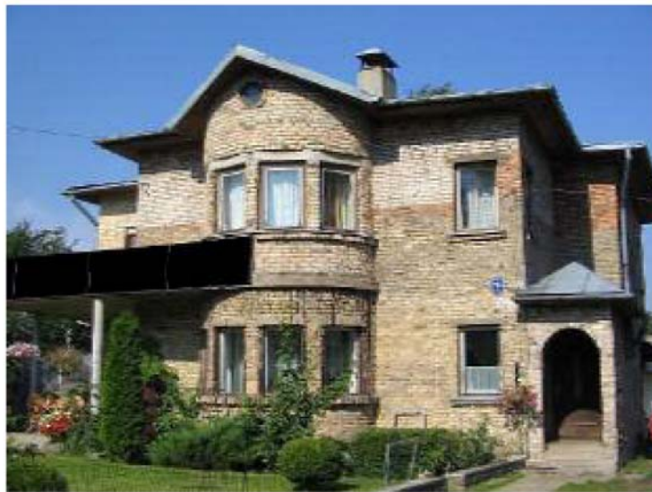
Figure 9. Photomontage illustrating balcony fence integrated solar collectors.
