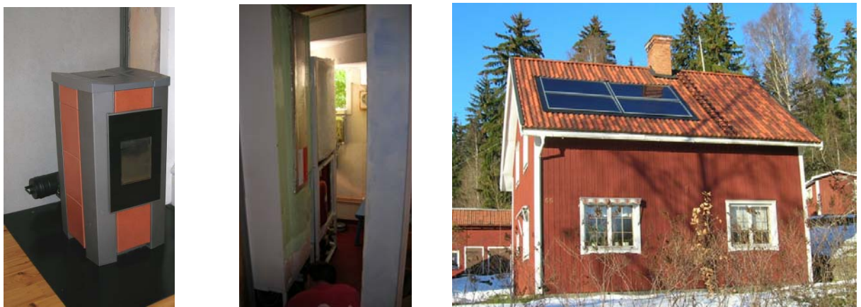
Figure B-3: The demonstration site in Borlänge, with (left) water jacketed stove, (middle) technical and store units in a cupboard under the stairs, and (right) view of the 10 m 2 collector array on the roof.
