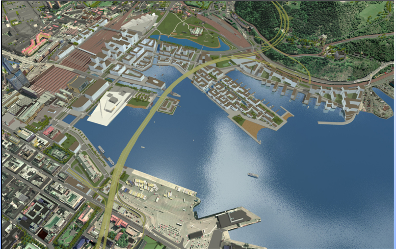
Bjørvika Concrete Tunnel
