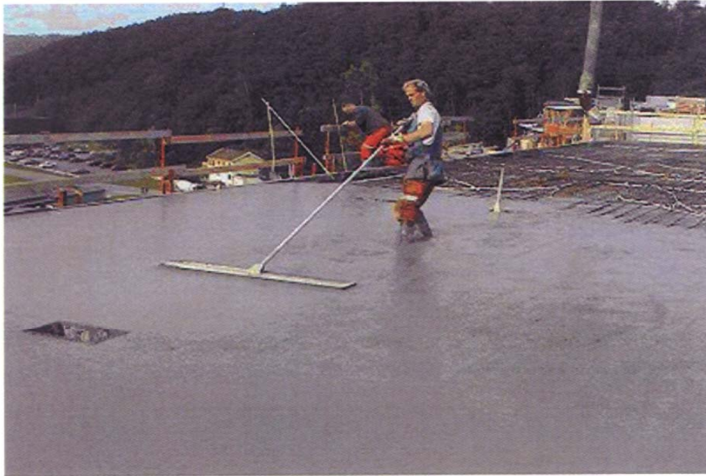
Figure 11.1 Levelling SCC with a skip float
