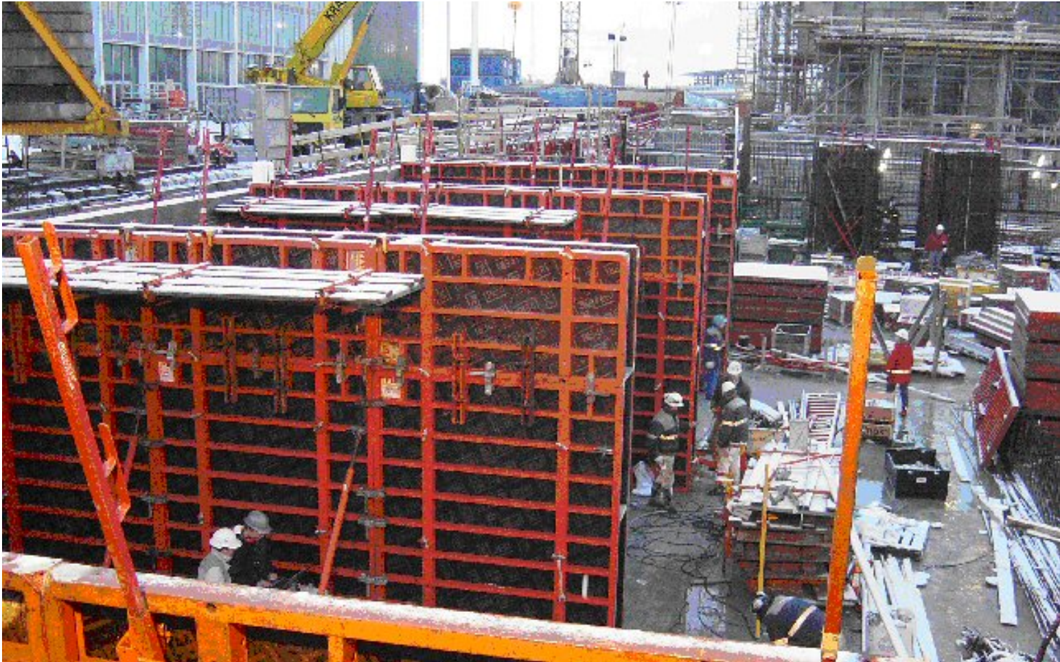
Ready for casting the three first walls of the basement in DR-Byen, Segment 3.
