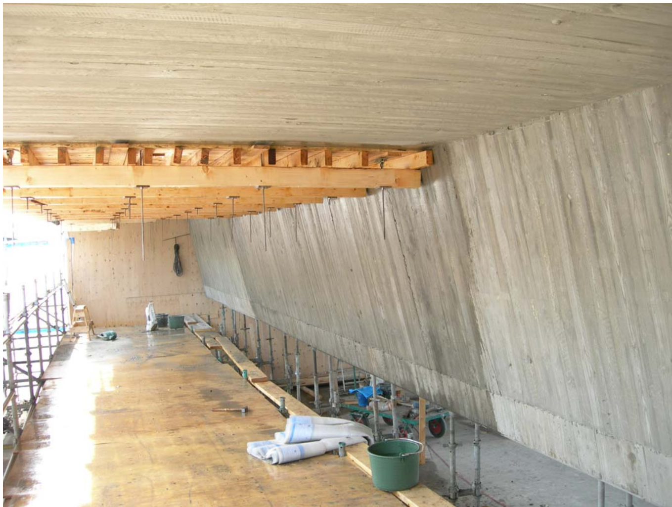
Part of east console and beam
