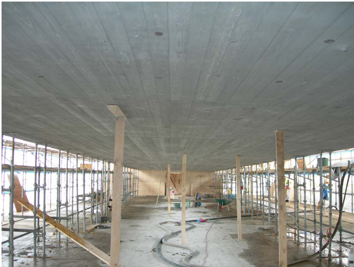
Finished bottom of beam
