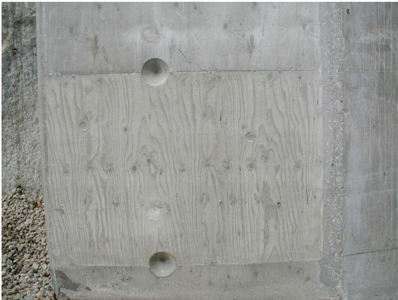
Detail, surface cast against Plywood
