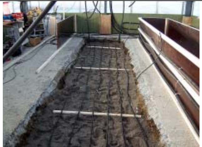
Sandlager under betongulv
