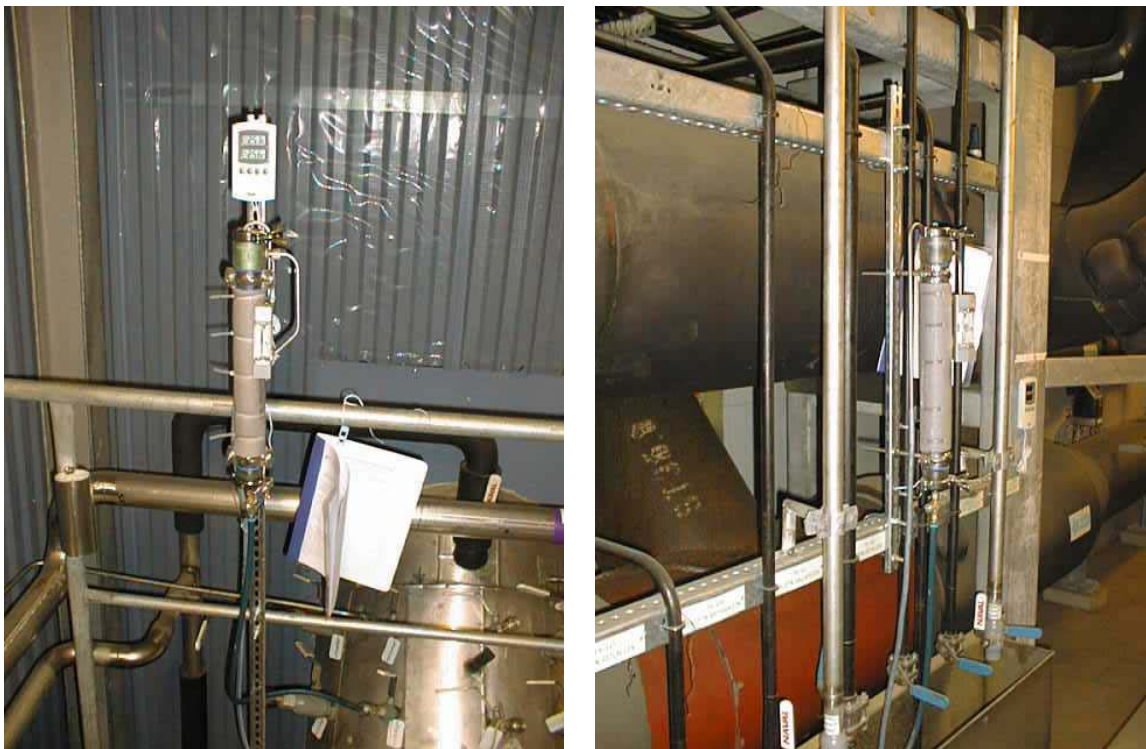
Fig. 4.5.3. Examples of locations for connection of exposure containers. The picture to the left is from the net at Värtan and the other picture is from the net at Solna. The exposure containers are covered with a foam plastic case for avoiding possible interference from surrounding light. Beside the exposure containers is a notebook for regularly notifications of the temperature and the flow of the district cooling water.
