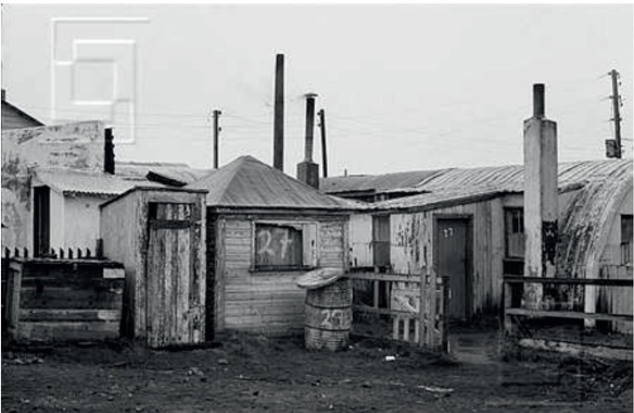
Figure 3. Kamp Knox in Reykjavik in the post WWII period (source: Ljósmyndasafn Reykjavíkur 2013)
