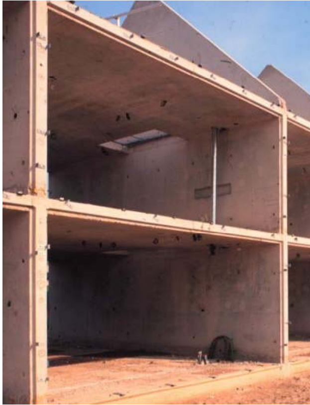
Figure 16. Concrete floor and wall edges shaped when casting with tunnelform to facilitate the sealing around the wall panels. Horizontal section in top detail and vertical section in bottom detail. Source: Ref [4] (photo) and ref [5] (details).
