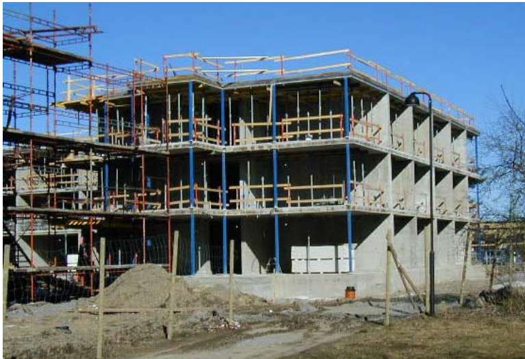
Figure 3. Multi-family housing structure of concrete and steel waiting for the in-fill timber frame exterior wall panels. Linköping, Sweden.
