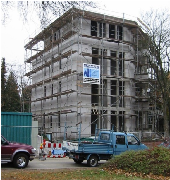
Figure 2. A typical 4 storey multi-family masonry building under construction in Darmstadt, Germany.
