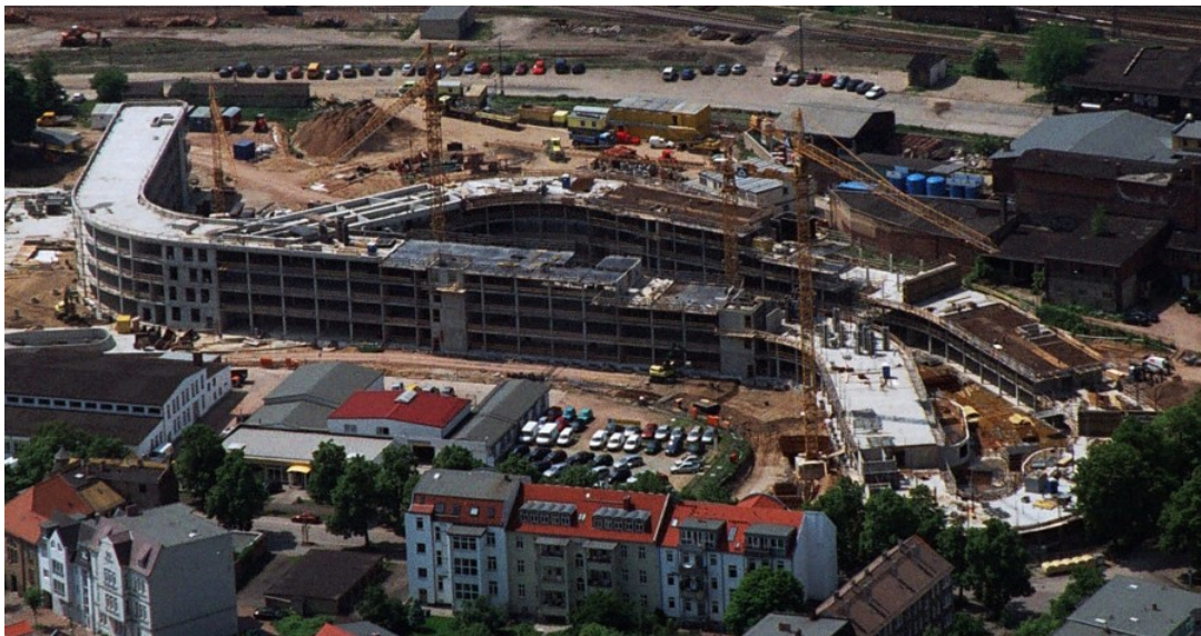
Figure 8. The construction site for the new German Ministry of Construction in Dessau. For a construction detail see also figure 11b. Source: www.umweltsbundesamt.de .
