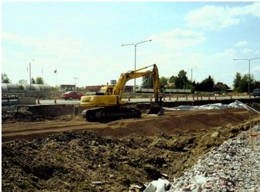
Figure 4.2 Construction work at Tuupakka Test field
