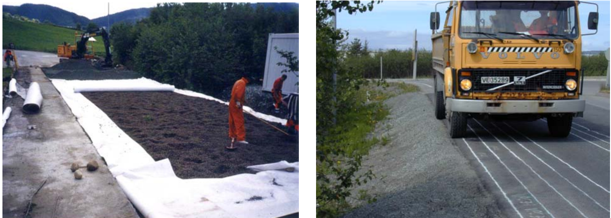
Figure 4.8 Sandmoen test field. Construction work and controlled loading test
