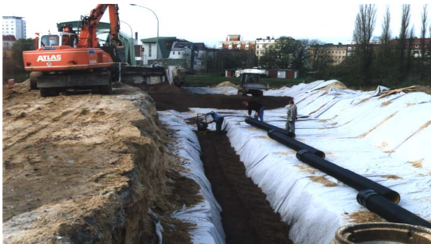
Figure 5.3 LWA in drainage ditch
