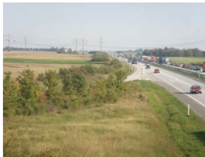
Figure 23. SRF as a wind shelter for snow protection along a motorway
