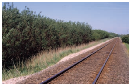
Figure 24. SRF along the railroad Malmö-Ystad
