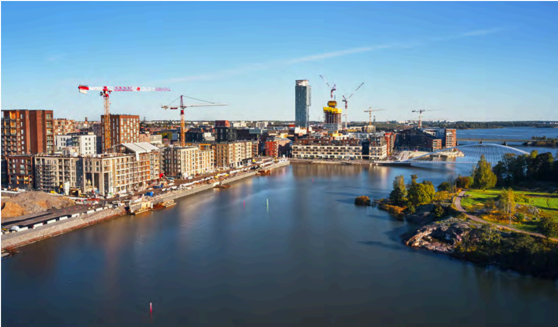
Figure 8. Construction in Kalasatama, a new waterfront area being developed in Helsinki
