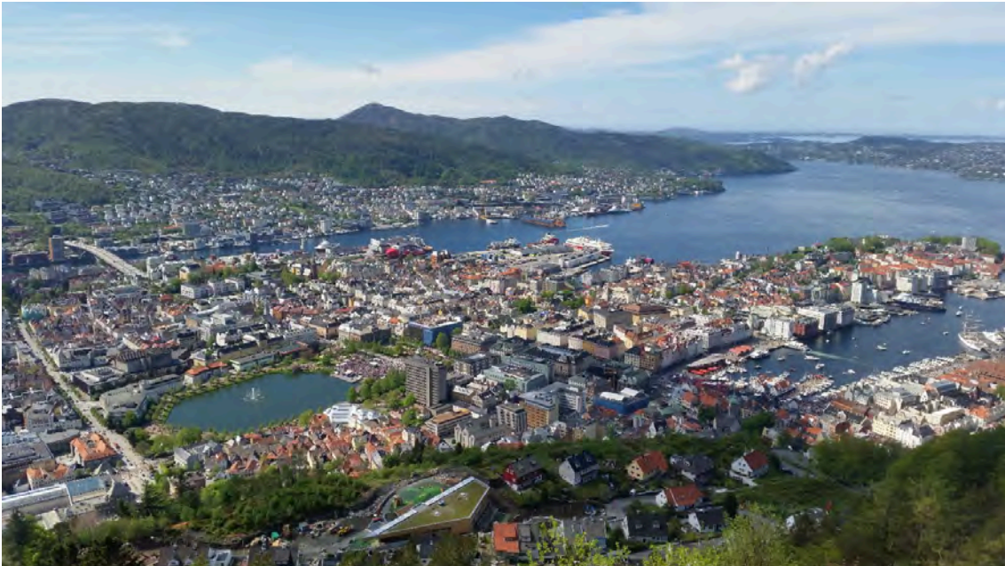
Figure 27. Aerial view of Bergen
