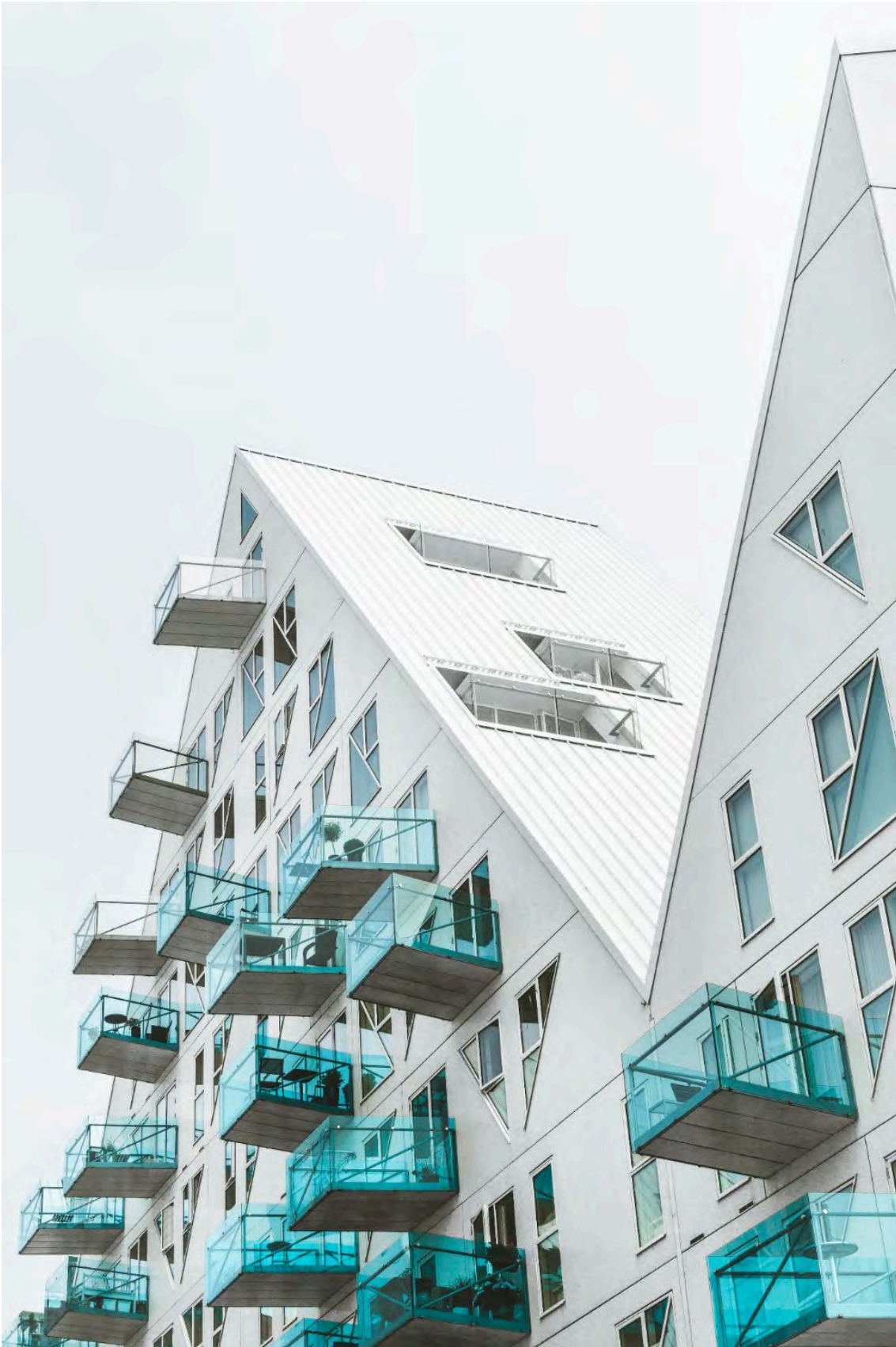
Figure 26. Aarhus Ø, an urban development site in central Aarhus on the city's former container port
