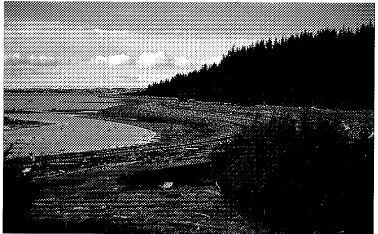
Figure 3.23 In the mid-1970s, a causeway was constructed over Svaet, a shallow area of sea (on average about 10 m deep) separating the island of Tautra from the mainland. It completely blocked the strong current that once flowed through Svaet and soon led to a build-up of sediment and changes in the production of marine invertebrates (bivalves, etc.) and other creatures. This transformation in the ecological conditions has brought about a marked reduction in the number of aquatic birds inhabiting the shallows, and the number of sea birds breeding on Tautra has also dropped dramatically due to predation from terrestrial mammals, such as mink, that have gained access to the island.
