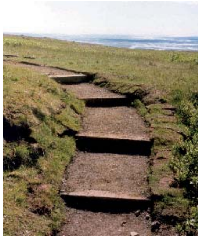
At Skaftafell erosion from traffic is minimized by the construction of footpaths (photos: Chas Goemans).
