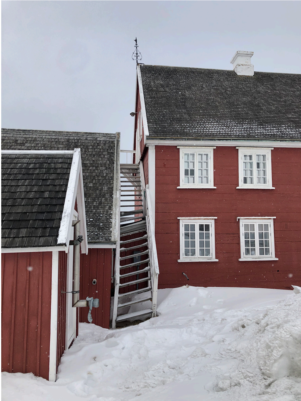
The High Arctic is considered particularly vulnerable to climate change. Climate adaptation of infrastructure and services is therefore particularly important in Greenland. The picture shows the effects of thawing permafrost on a building's stairs.
