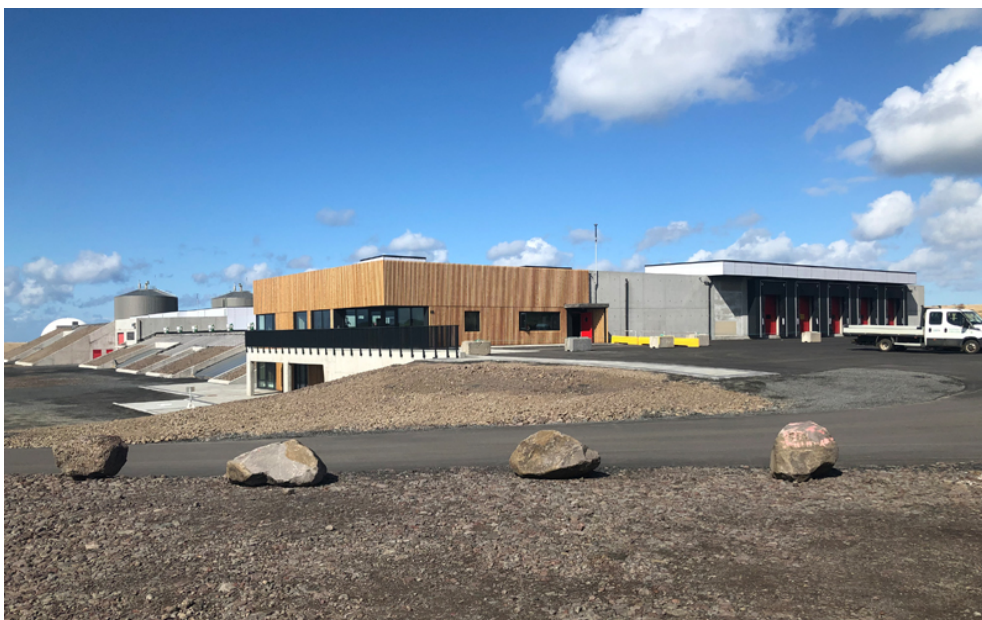
Figure 10: New biogas and composting plant (SORPA, 2020).
