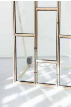
— Figure 12 Glass facade made from used glazed windows
