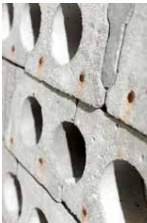
— Figure 75 Concrete bricks made from concrete slabs
