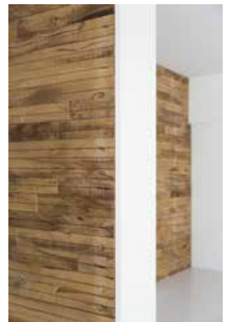
- Figure 9 / Dismantled floorboards from renovation repurposed as wall cladding, Vandkunsten in Albertslund Syd, 2014.
