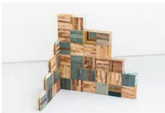
Figure 64 > Indoor wall made from used interior wood
