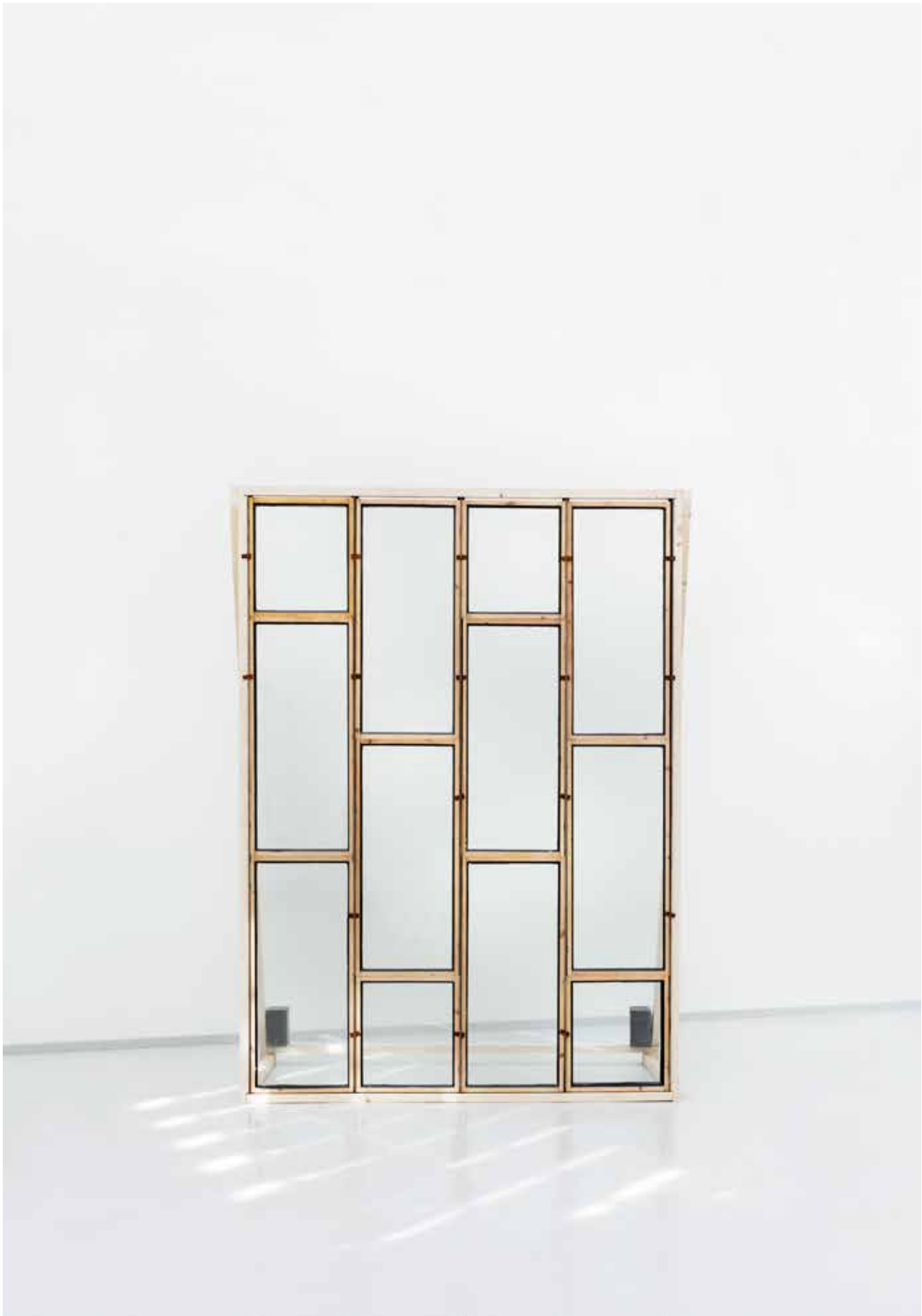
- Figure 35 Prepared window elements, a DfD detail and the assembled prototype of an interior wall from repurposed windows
