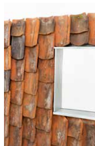
— Figure 77 Facade cladding made from roof tiles
