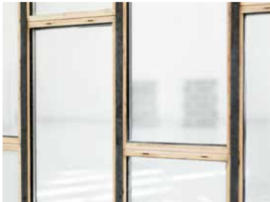
Figure 63 > Glass facade made from used glazed windows
