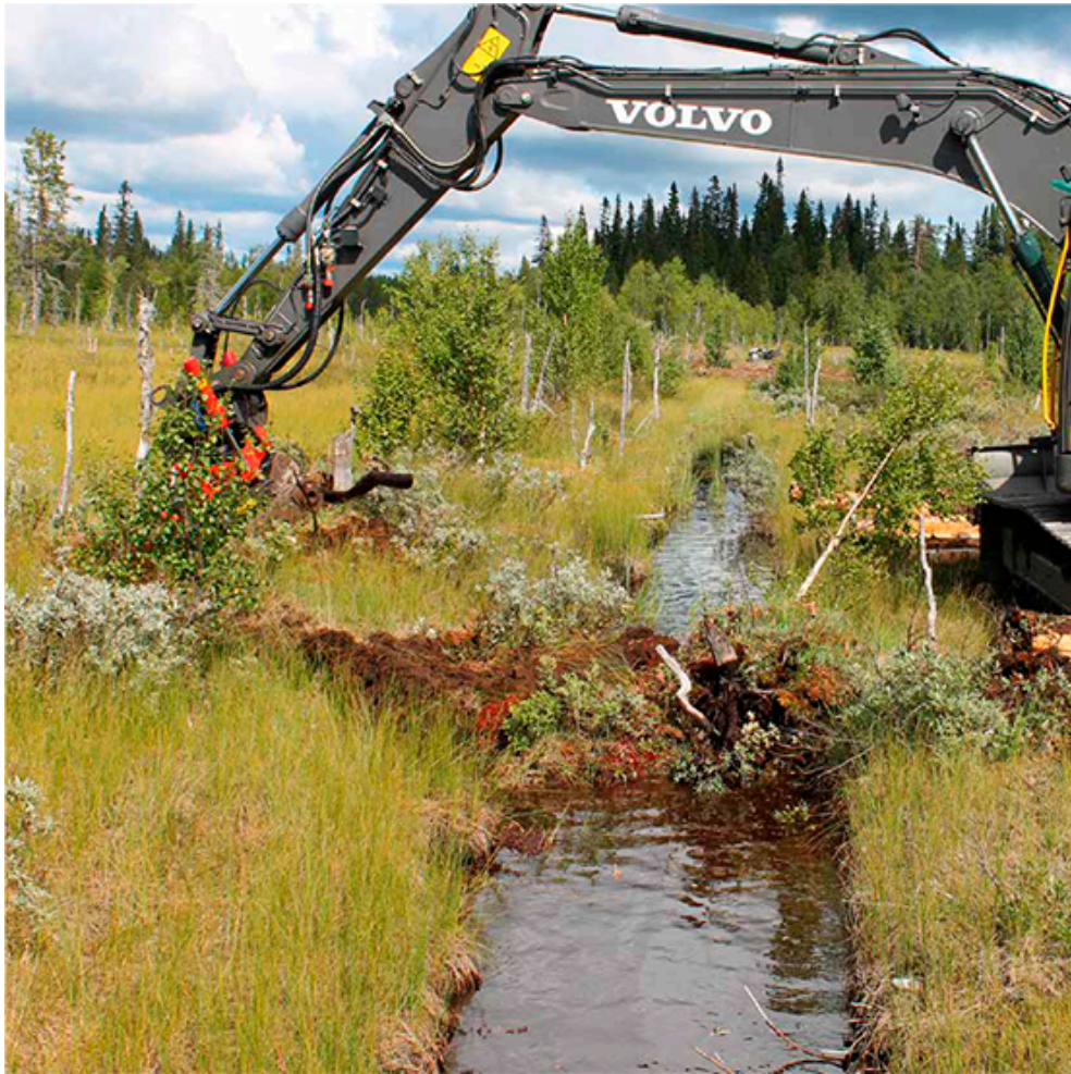
Fig 6.2.2. Excavator filling in a drainage ditch to raise the water level in a drained mire. Notice the invasion of trees along the banks of the canal where the ground is higher due to drainage. All-together more than 3,200 dams were established and in total, the project has restored hydrology in more than 2,800 hectares of drained mires, removed trees and shrubs in 1,800 hectares of overgrown wetlands, and restored 15 hectares overgrown wet meadows for renewed haymaking. Source: The EU LIFE to ad(d)mire project 2010–2015. Photo: Länsstyrelsen, Jämtland.
